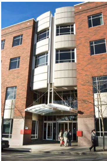
Entrance to one of the UWMC Roosevelt clinic buildings.
