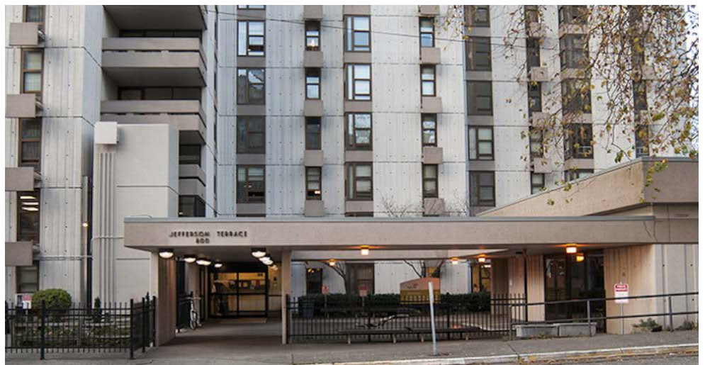
The entrance to Edward Thomas House Medical Respite on Jefferson Street
